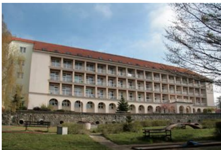
Rehabilitation institute Kladruba
